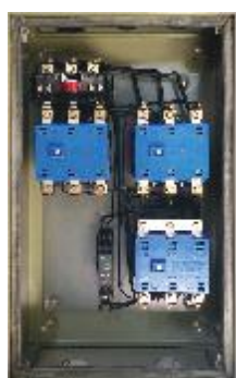
Interior View of ML FASD
