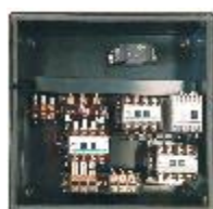
Interior View of MU-G20W FASD
